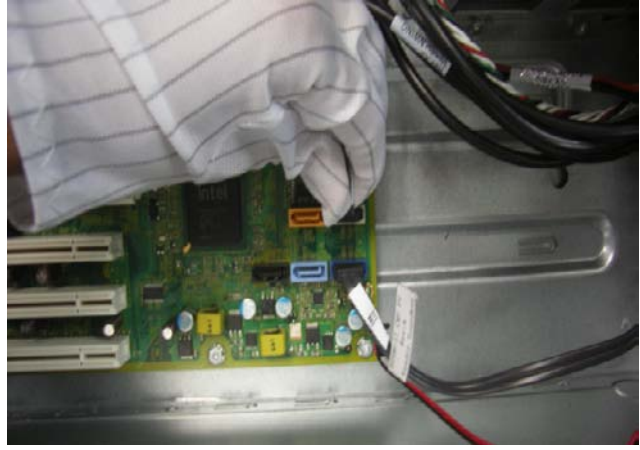
Figure 2 Disconnect the cables from the board
