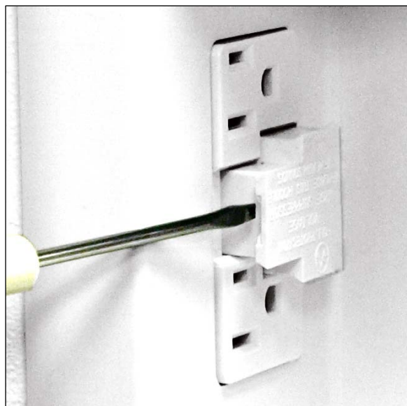
Removing the SurgeBloc® Module
